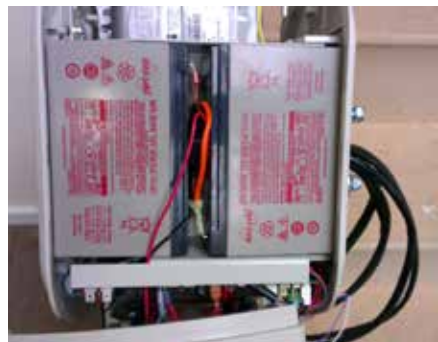
BATTERIES ROTATE BACK IN PLACE
