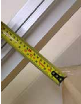
RAIL TO STEP NOSE MINIMUM OF 3 1/4"
