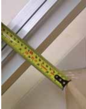
RAIL TO STEP NOSE MINIMUM OF 3 1/4"
