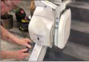
Attach bottom cover of drive train .
